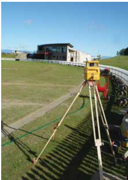
A collector drain was installed right around the cricket ground
