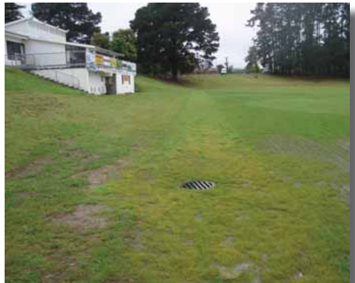
The new swale drain and sump at Waikanae Park
