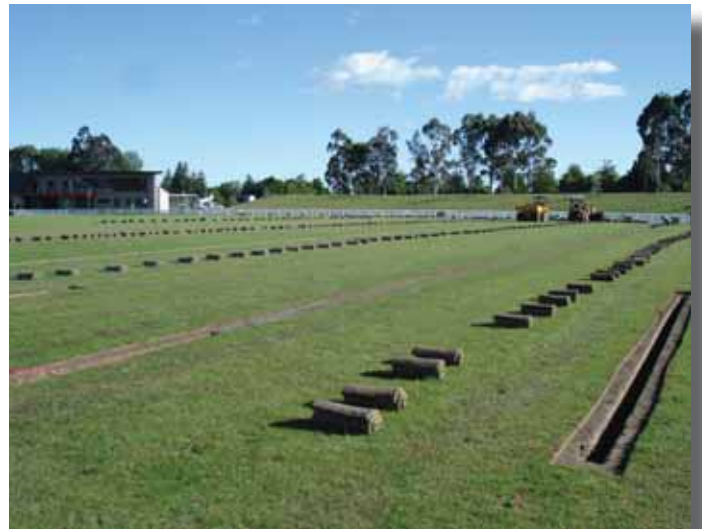
Turf is rolled away as trenching work begins
